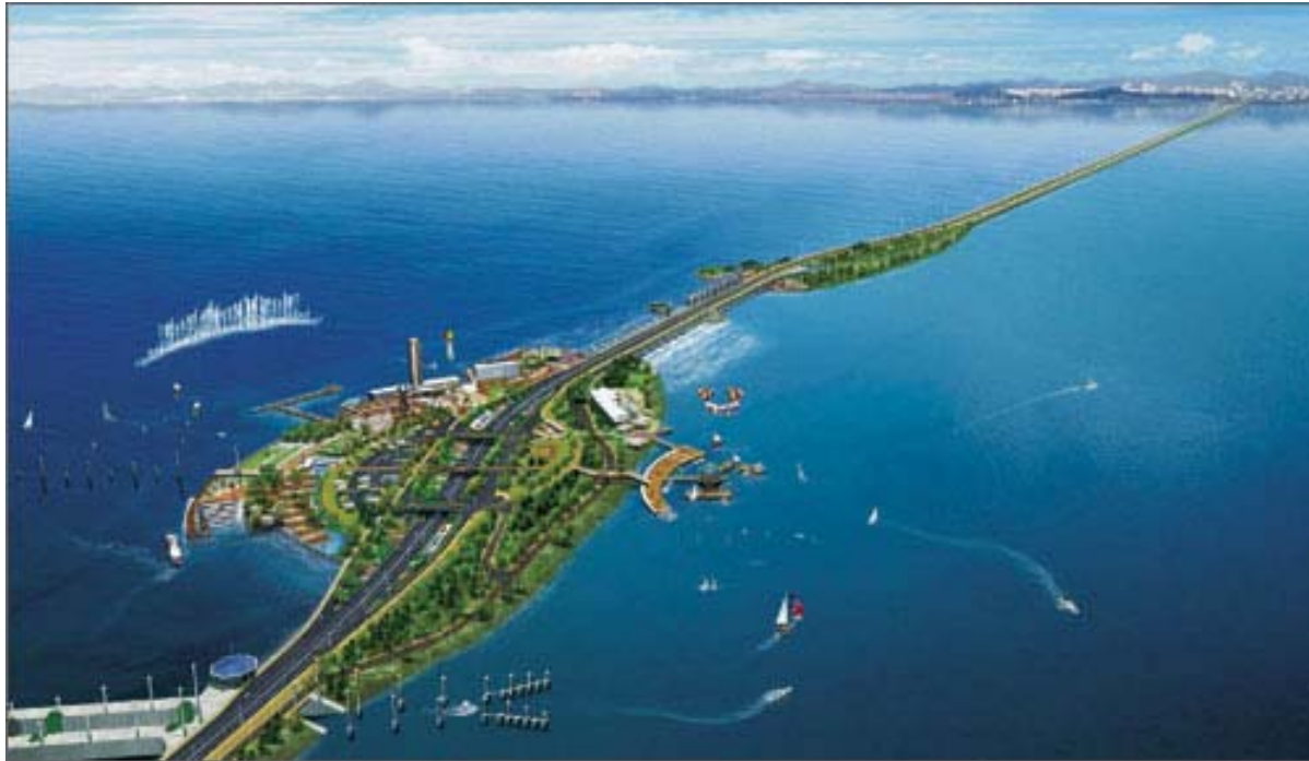
Sihwa Tidal Power Plant in 2009
